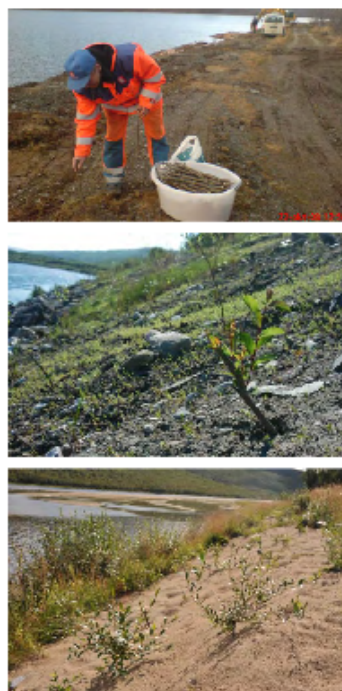
Figure 11. Planting catches down by the propagation. The catches are being prepared in the ground and are based on the spreading of the soil in small patches of yellow soil to create a better local soil conditions. Photo: Sørensen, NVE.
